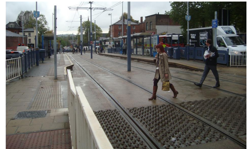
Sheffield: staggered crossings, harsh surface
