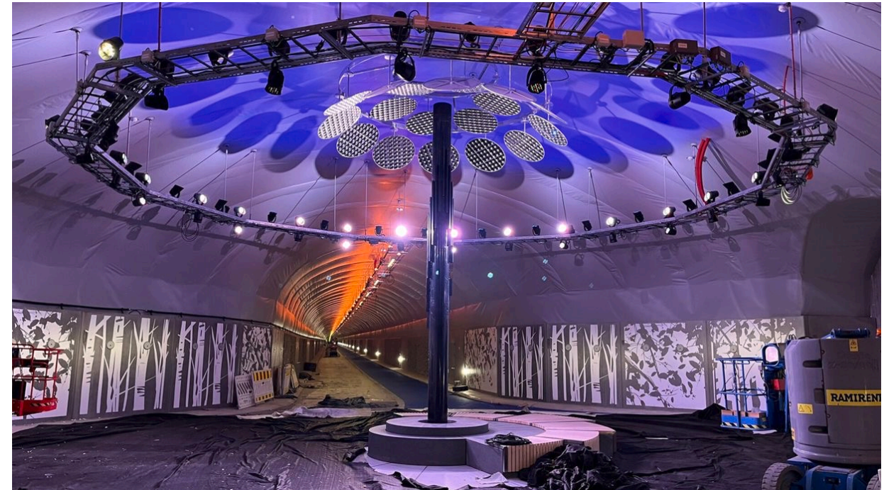
Rest area in the middle of the tunnel
